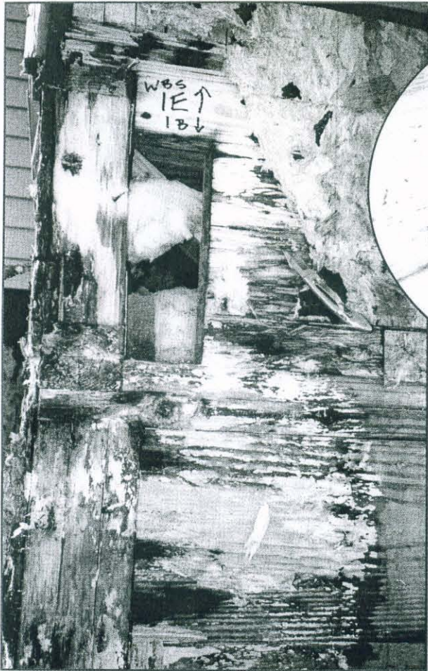
Photos 6 and 7 show water-damaged building components caused by improper waterproofing details at a deck. These buildings were clad with wood siding.
