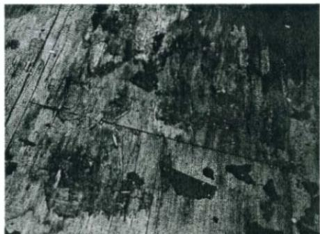
*Damage from moisture intrusion also ruined vast expanses of the plywood roof decking, which had to be replaced.*
