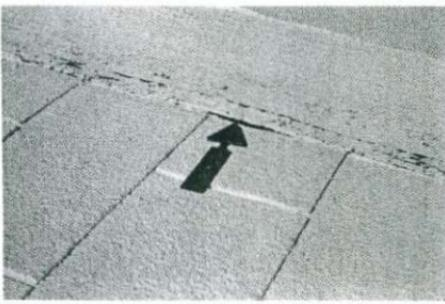
*The old roof shingles are covered here with an elastomeric coating. The arrow points to a gap in the roof which allowed moisture to penetrate and corrode metal flashings.*
